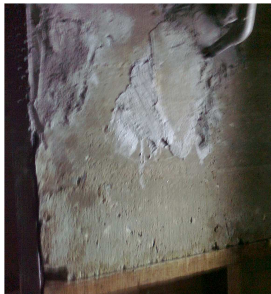
(B).Application test in pasting and grouting
