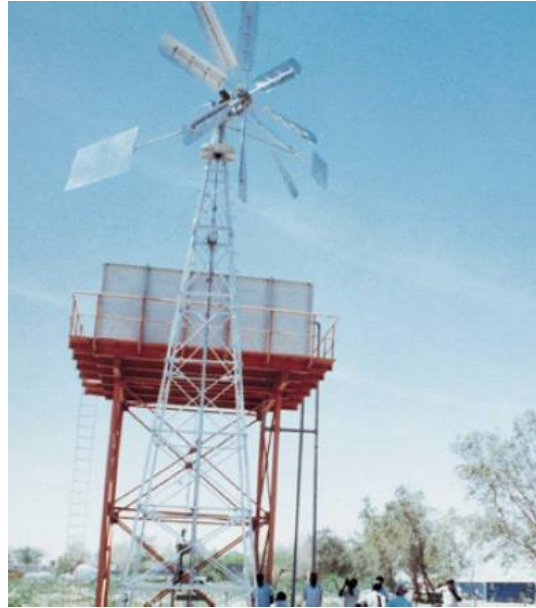
Figure 5. Locally-manufactured wind pump installed at kilo 8 site
