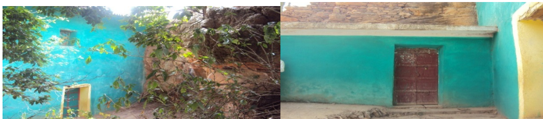
Figure 13. The modern church of Enda Abel built within the ancient Cave church. The tomb of the Saint Enda Abel, Mai Ambessa Hamlet Degou
